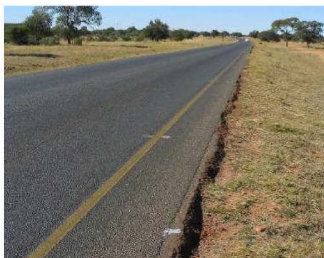
Photo 4-2: Botswana example of low volume road constructed with laterite base course
